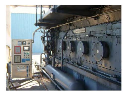
of the old air-operated vibration switches. They decided to replace the old system with the Altronic VSM monitor. They also updated the waste gate controller with a cable-driven Moore that is controlled by the PID loop on the DE-3000.
