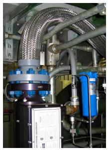
Flexible fuel line installed
