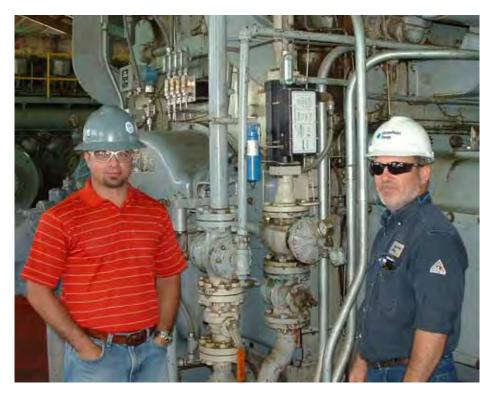
the needs of our unit. After the first governor was installed, our team installed the other two GOV-50's and the GOV-10. We copied the program from the first unit and used it for the others. The only obstacle encountered was with one of the analog out circuits that allows us to read engine speed. It was resolved by simply removing the cover and cutting a jumper wire.
