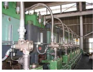
Cam actuated start valves with pressure-actuated in-head check valves
