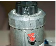
**Zero Governor** The zero governor will have a seal applied from the regulator adjustment screw to a hole in one of the support braces.
